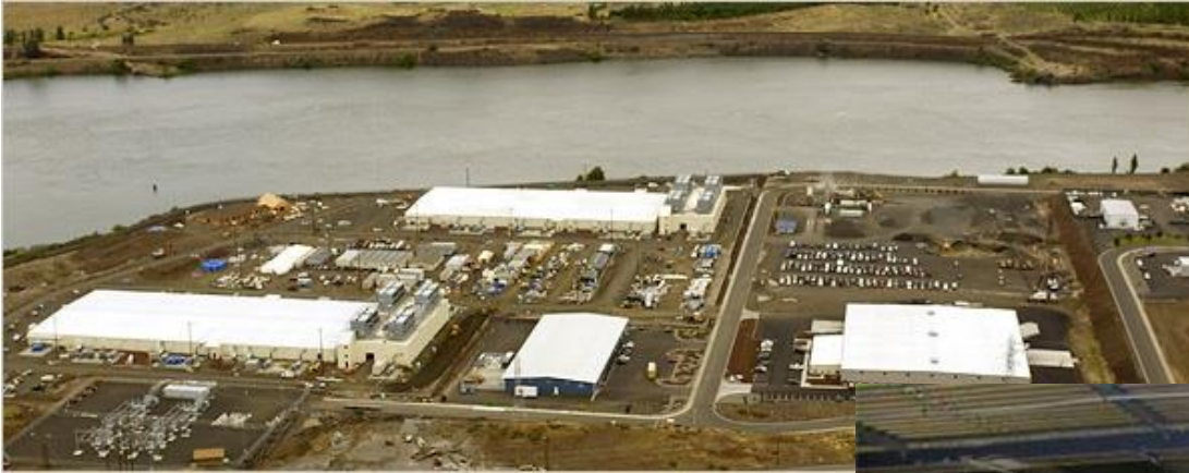
Google's Datacenter in Oregon
