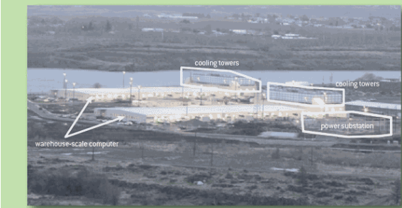
FIGURE 1 An Example Data Center and Warehouse-Scale Computer
